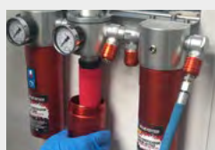
1. Unscrew lower section
