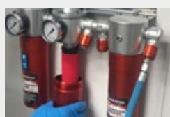
1. Unscrew lower section
